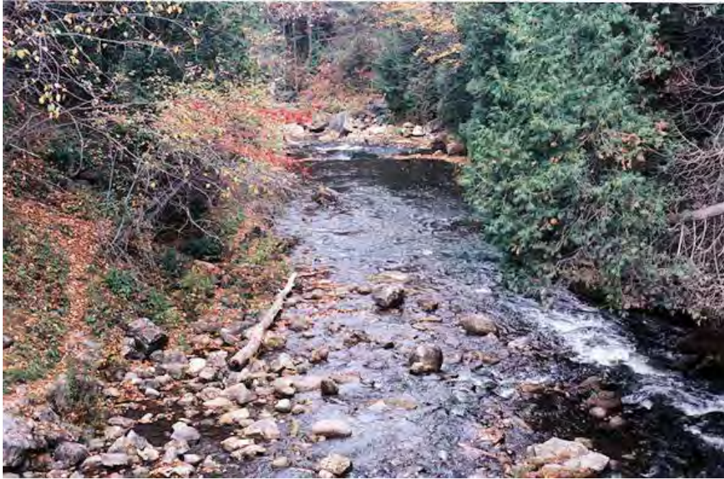
Figure 3.3.2: B - Type Channel, looking downstream from the Belfountain Dam*
