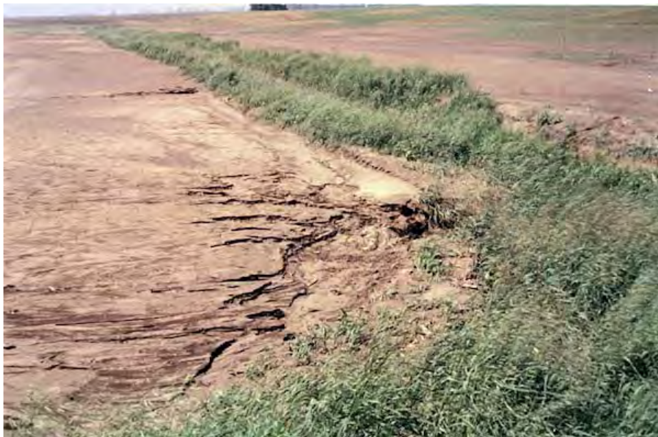
Plate 4. Ground view of erosion along a drain in the Rondeau Bay watershed, June 4, 1981.
