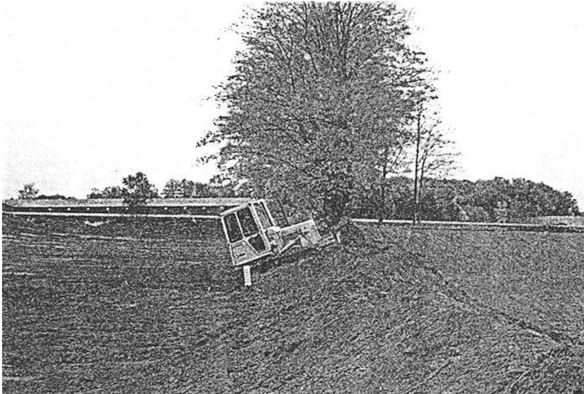
Fig. 11: WASCOB Construction on the McMurray Property.
