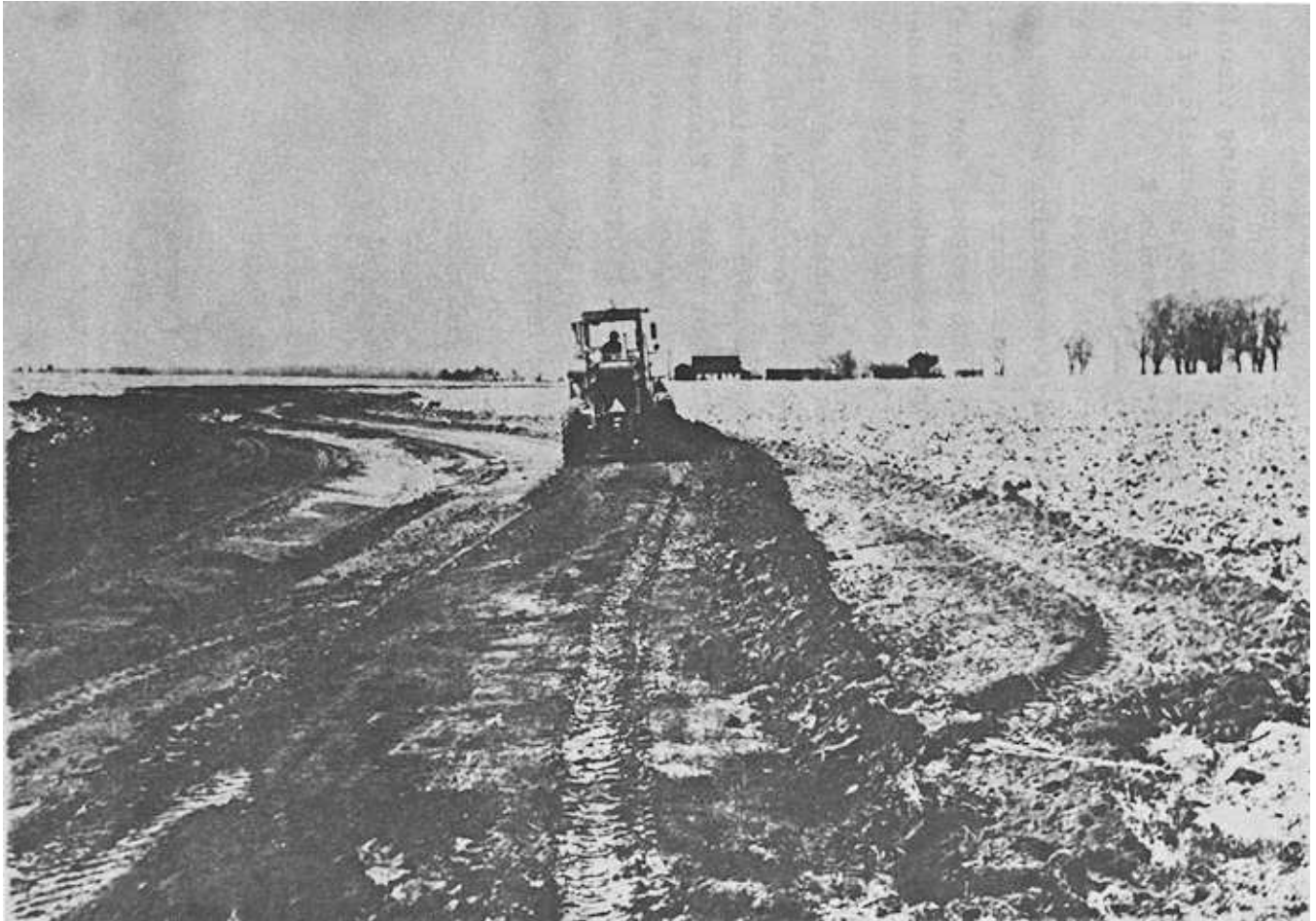
Figure 4. Grassed Waterway Grading
