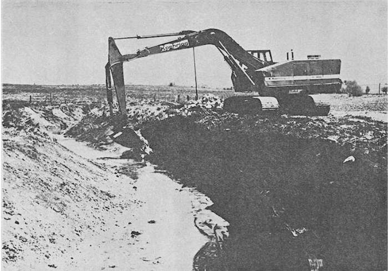
Figure 5. Municipal Drainage Work
