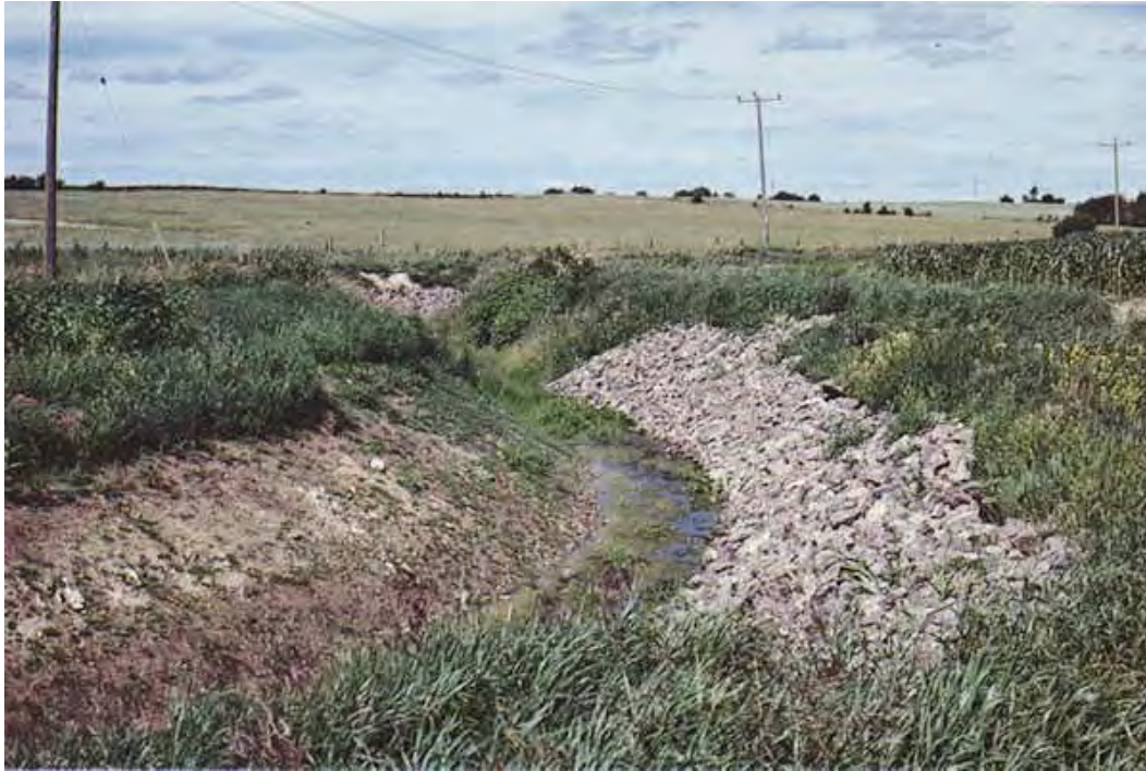
Figure 9. Proper Drain Construction
