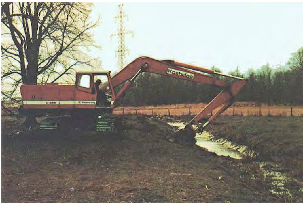
Figure 10. Regular Drain Maintenance
