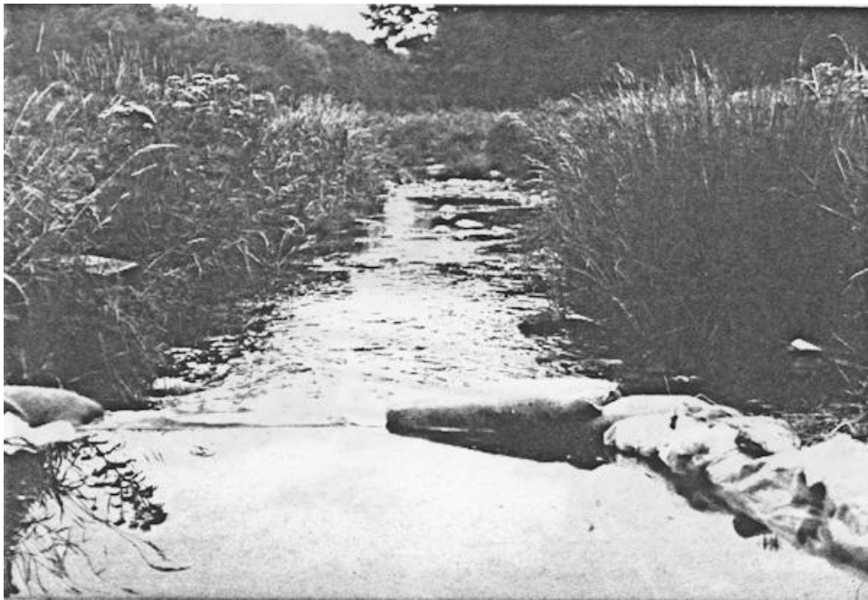
FIGURE 6: LOOKING DOWNSTREAM OF THE 3-STEP DESIGN WEIR
