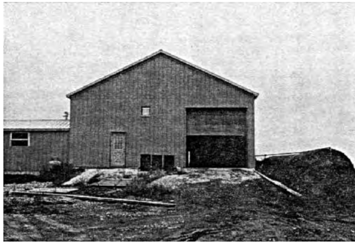
Figure 5. An overview of the Gasser digester with farm shop/cogeneration building and flexible biogas storage protection tank
