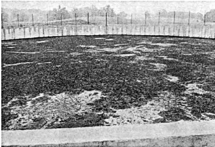
Figure 21. This is raw dairy manure held in a tank prior to land application. Note the scum buoyed by gas production in the tank
