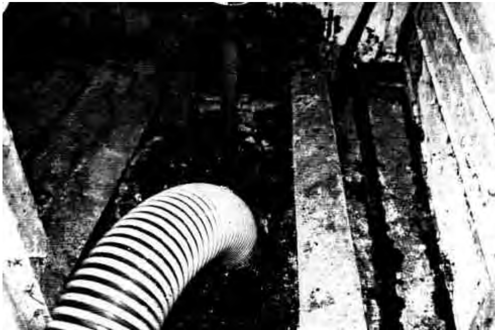
Plate 2. Sump pit at the swine farm.
