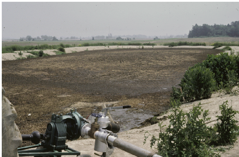
Figure 1 Earthen manure storage during pump-out
